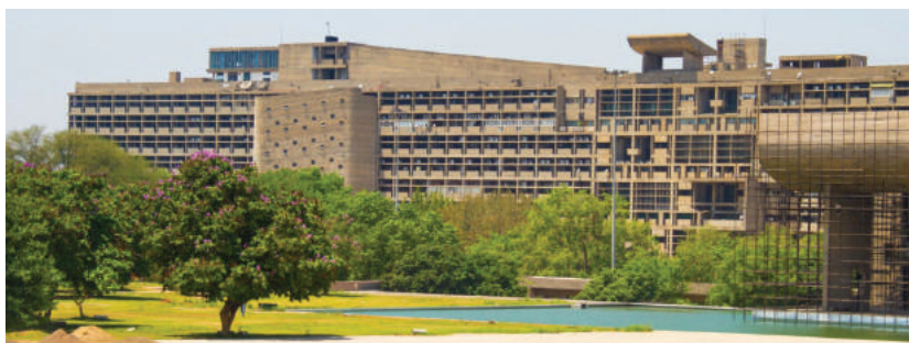
The 240m high Secretariat was the tallest building in Punjab when it was built.
